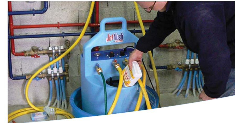
System flushing equipment
